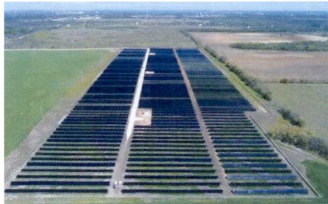
▲ Highway 56, Sherman Texas, 7.2 MW
