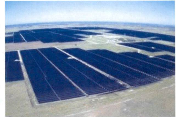
▲ Wagyu Solar, Damon Texas, 162 MW
